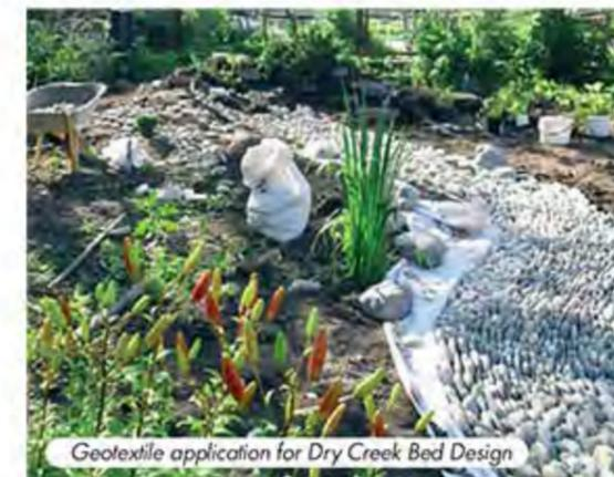
Geotextile application for Dry Creek Bed Design
